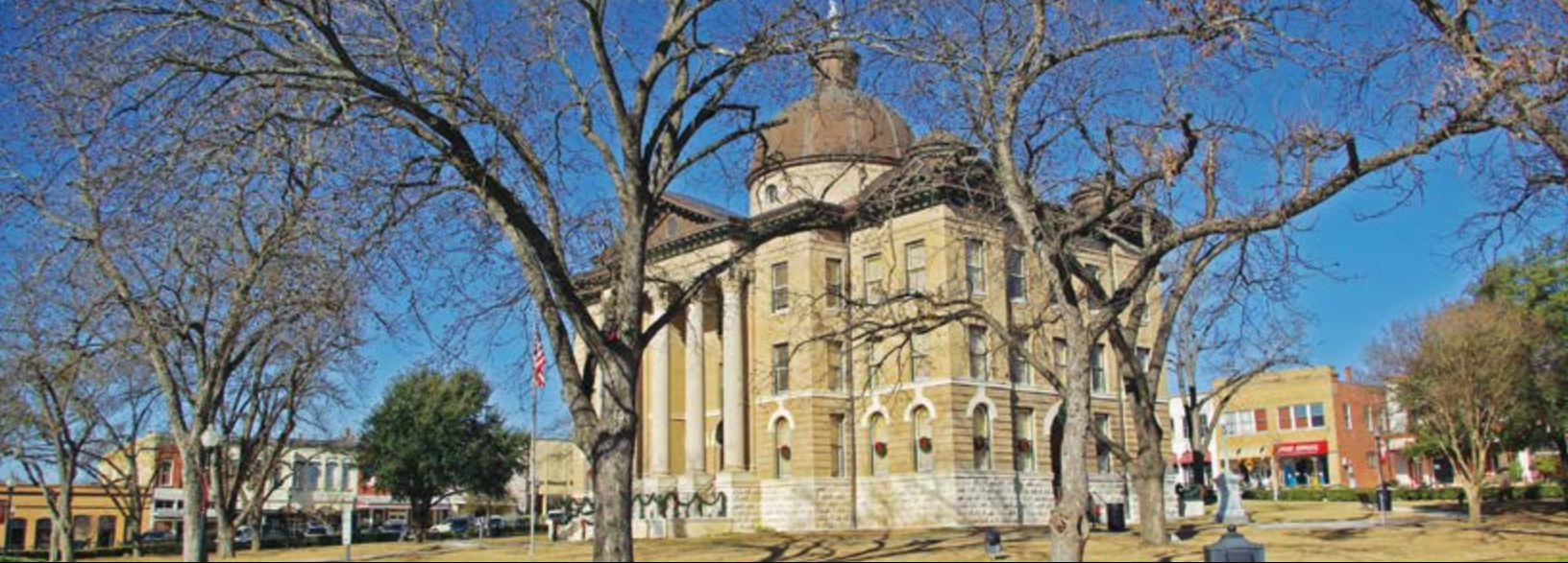
Hays County Historic Courthouse
